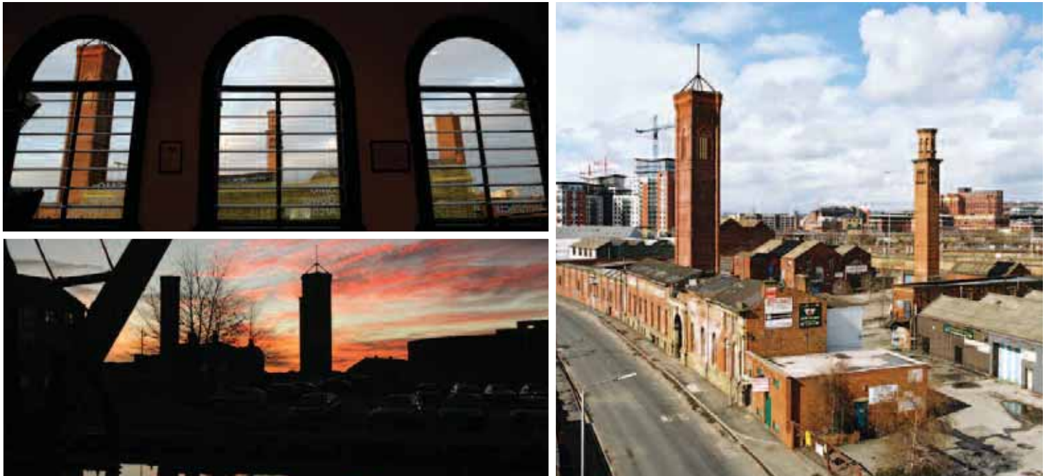
Views of Tower Works
