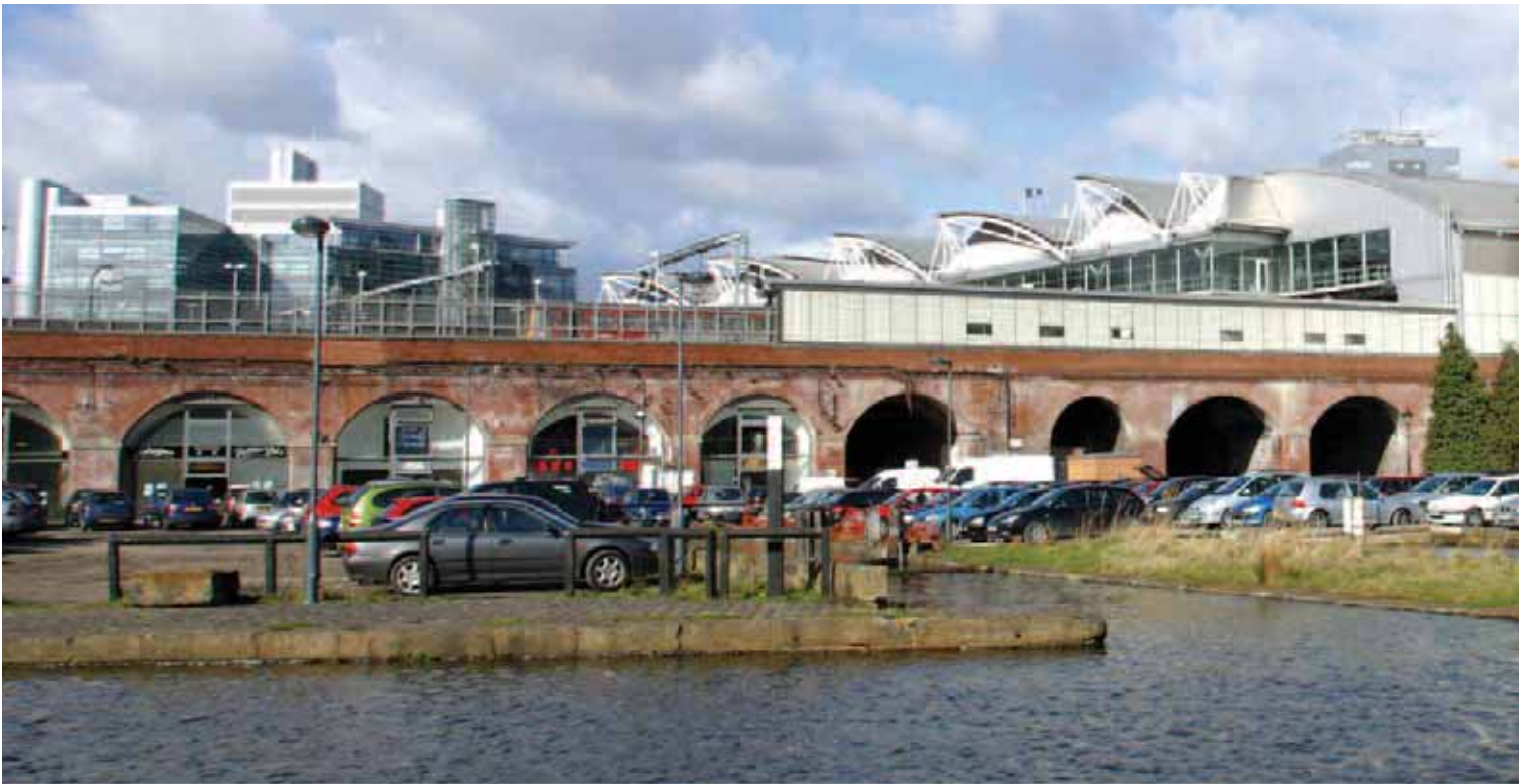
Car parking at Granary Wharf
