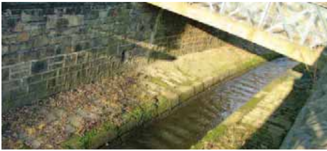
Much of Holbeck Urban Village area lies within a flood plain identified by the Environment Agency.
